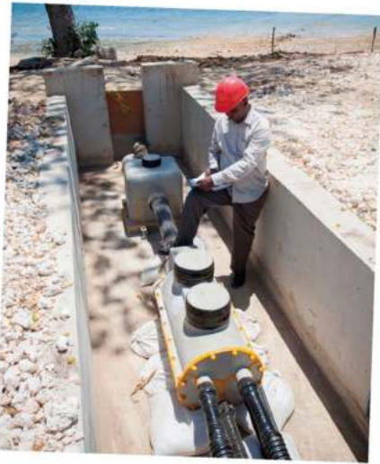
Testing an undersea power cable on the beach in Zanzibar
