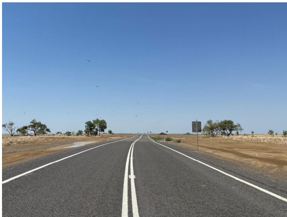
Image: Courtesy of the Department of Transport and Main Roads — Queensland Richmond-Winton Road upgrade.
