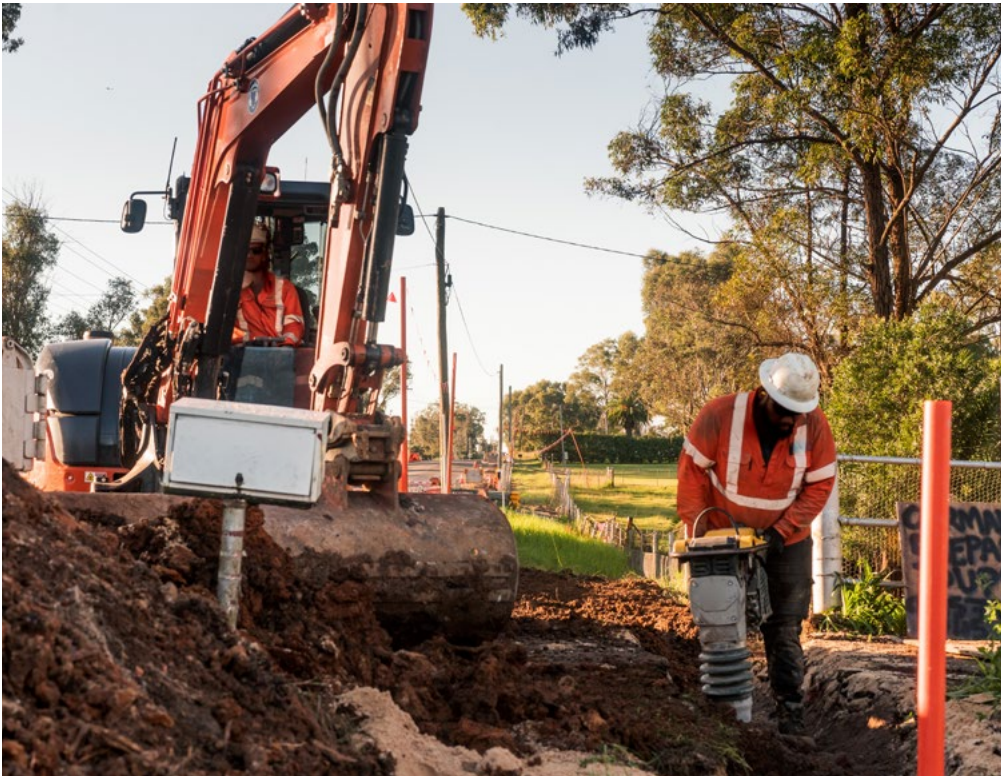
Image: Construction worker soil stamper with digger. Credit: DITRDCA
